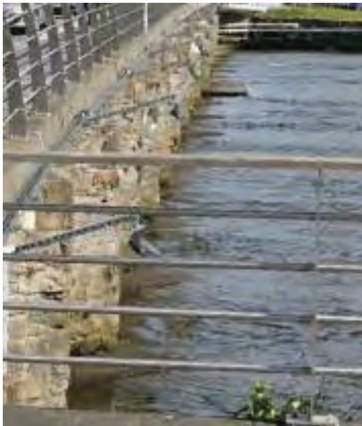
Figure 5.12: Lighting illuminating Arches on Arklow Bridge
