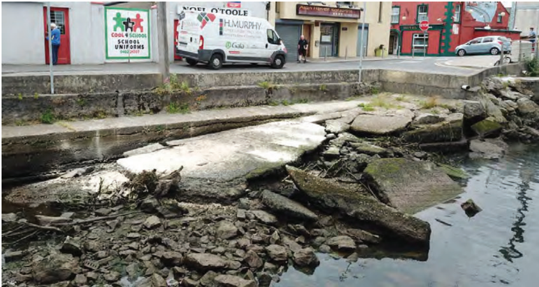
Figure 5.9: Location of RA7 at Coal Quay slip
